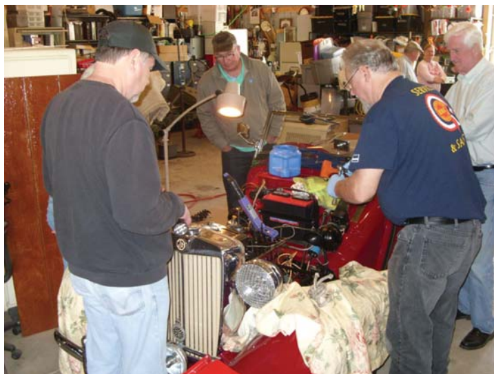
Jim Pesta (in the blue T-shirt – an appropriate attire for the day) prepares to compress the valve spring on Steve's TD. Note the purple custom-made spring compression tool..
